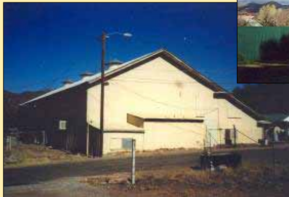
Trolley car Barn-Service Shed, Ariz. Public Service Co.
