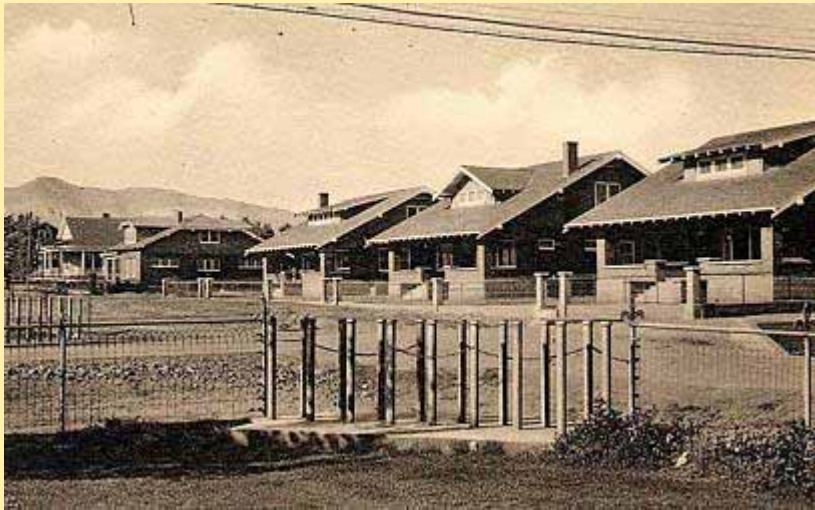
Craftsman bungalow style residential cottages were chosen as the unifying architectural theme to line both boulevards of Vista Park.
