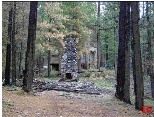
**Photos 15,16—homes destroyed adjacent to homes survived indicates that significant differences existed in the fire and home characteristics necessary to meet the requirements for home ignition.**
